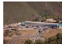
BT239 - NAVE INDUSTRIAL
